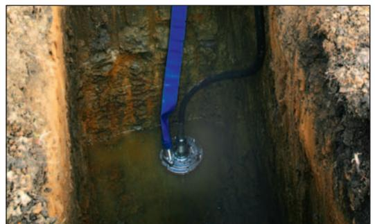
The shaft driven pump quickly empties flooded bunkers, trenches or graves with no priming.
